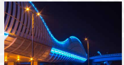
Architectural outdoor lighting
